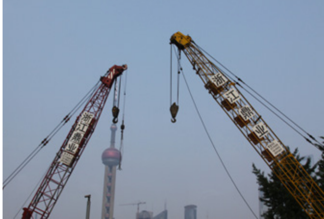
Cranes meet tower. Photo: Hsing Wei
