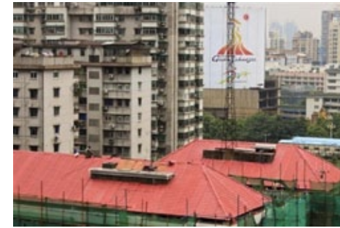
In the summer of 2010, the Guangzhou municipal government augmented the flat roofs of old apartment buildings with PVC boards so that passers-by would be given the illusion that they were sloped, red-tiled roofs. Source: Singsupplies.com
